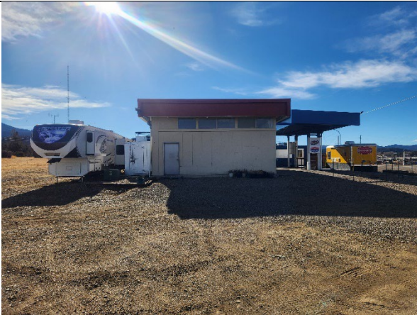
01. Looking south at the north site building.
