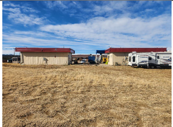
08. Looking west at the rear of the site buildings.
