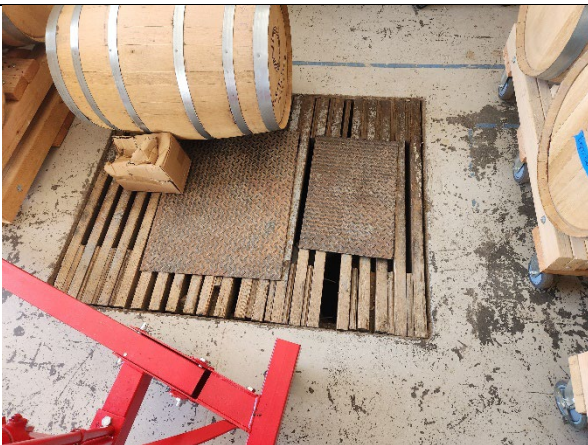
17. View of former sand trap in the north site building.
