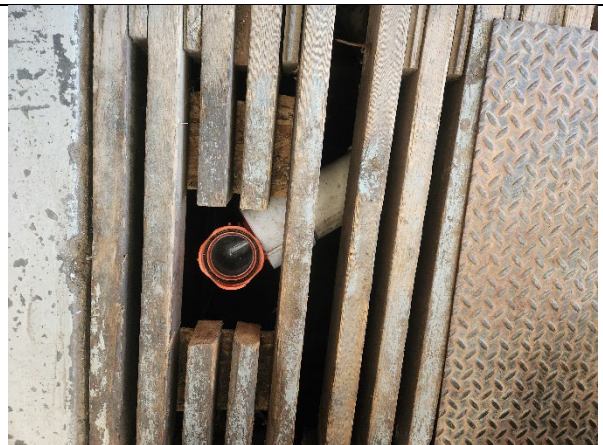
18. View of sanitary sewer connection in the former sand trap.
