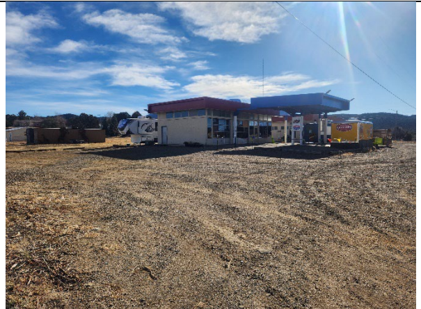
02. From the northwest corner of APN #12110000, looking southeast at the subject property.
